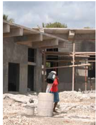
Rebuilding the School
