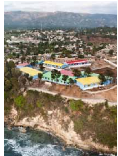
Aerial View of Completed School
