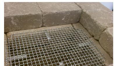
IMG 6: Install Spark Arrestor at top of fireplace stack.
