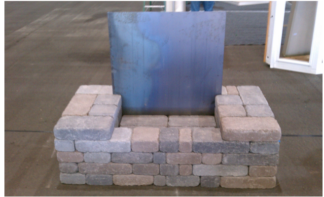
IMG 1: Metal Back-Plate Installed
