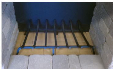
IMG 5: Place log grate on top of the fire brick.
