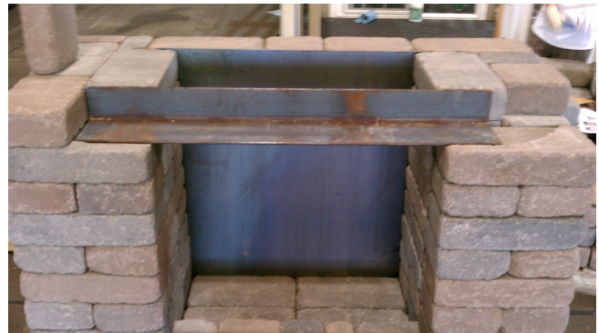
IMG 3: Lintel Placed in Grooved Unit and spans across opening
