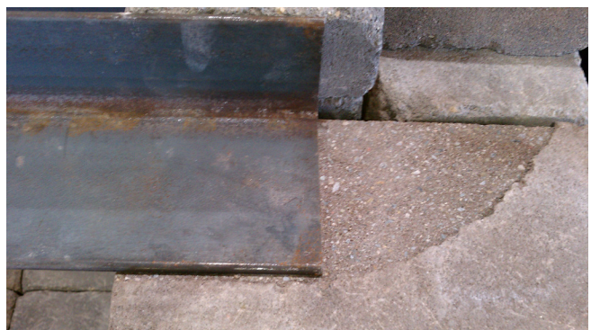
IMG 4: Lintel Placed in Grooved Unit - Close-up
